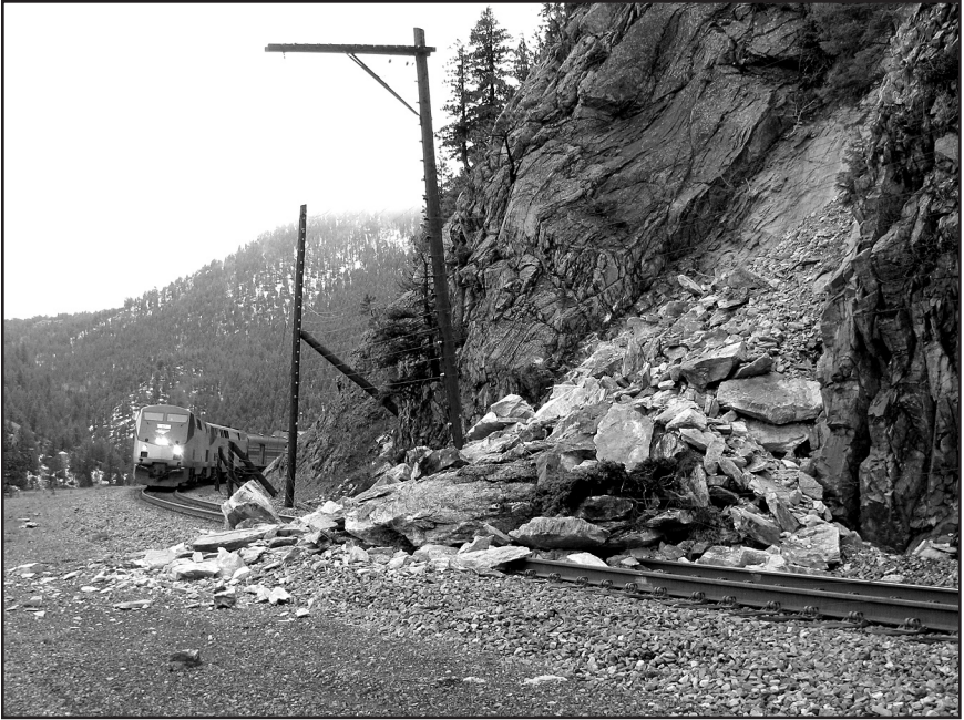
A rock slide through the slide detector fence on the Moffat subdivision on Saturday, May 15, 2010.
