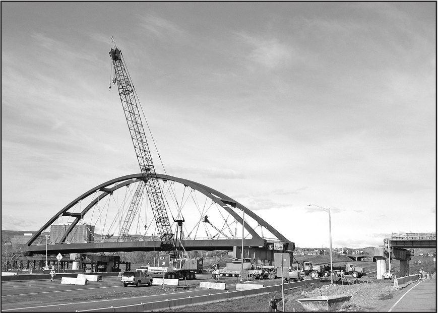
Denver's Regional Transportation District moved its West Corridor bridge over 6th Avenue on May 3, 2010. – Photo © 2010 Dave Schaaf.
